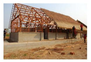
**9 Boarding Girls 1.** Finished the complete roof structure and started thatching ( $\uparrow$ ). Continued with interior masonry up to ring beam level. Ring beam has been shattered, reinforced and poured ( $\downarrow$ ).
